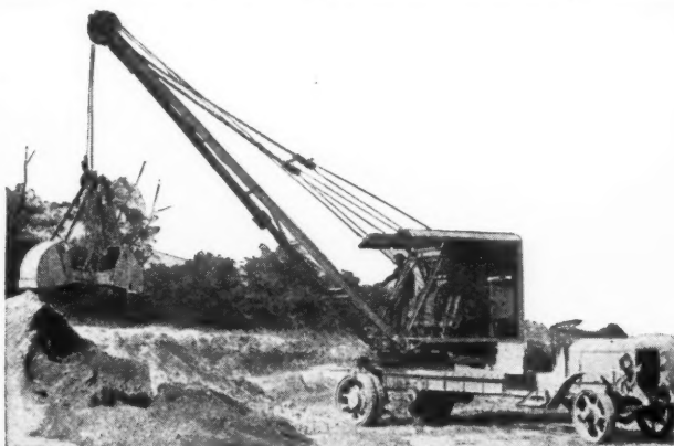
The New P. & H. Truck and Trailer Crane
